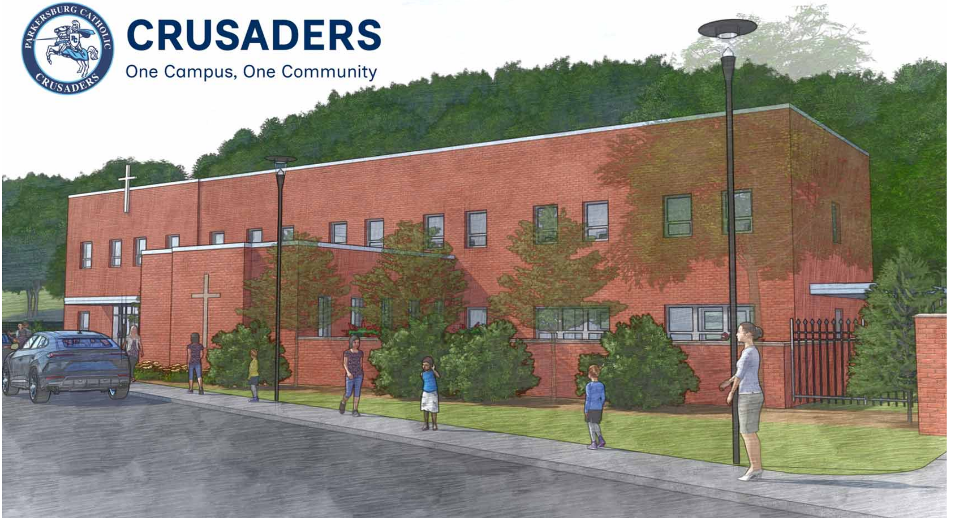
Courtesy of Pickering Associates
